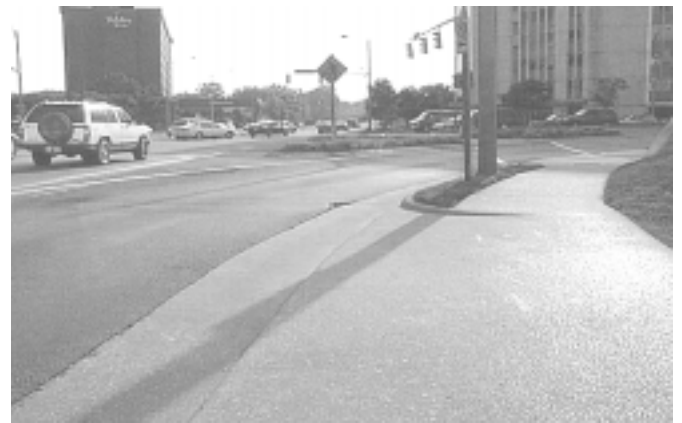
Pictured above is the free right turn lane on Fairfax Dr. at Glebe Rd. looking west at the north side of the intersection. The crosswalk is not readily visible. It does not have high visibility pavement striping and is also partially obscured by a sign and utility pole. There are no warning signs for motorists, although a “YIELD” sign is posted on the other side of the crosswalk. This location has proven particularly hazardous for neighborhood residents with disabilities who regularly cross at this location. Those crossing Glebe Rd. at this intersection have a pedestrian signal that flashes 7 seconds “walk” and 27 seconds “don’t walk” requiring a person on foot to cross the 100’ walkway in 34 seconds.
